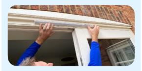
The distance between the clips isn't critical as they can fit on anywhere along the length of the aluminium part of the light. To mount the light simply fit one edge into the top or bottom of the clips then twist it round until it clicks into place.
